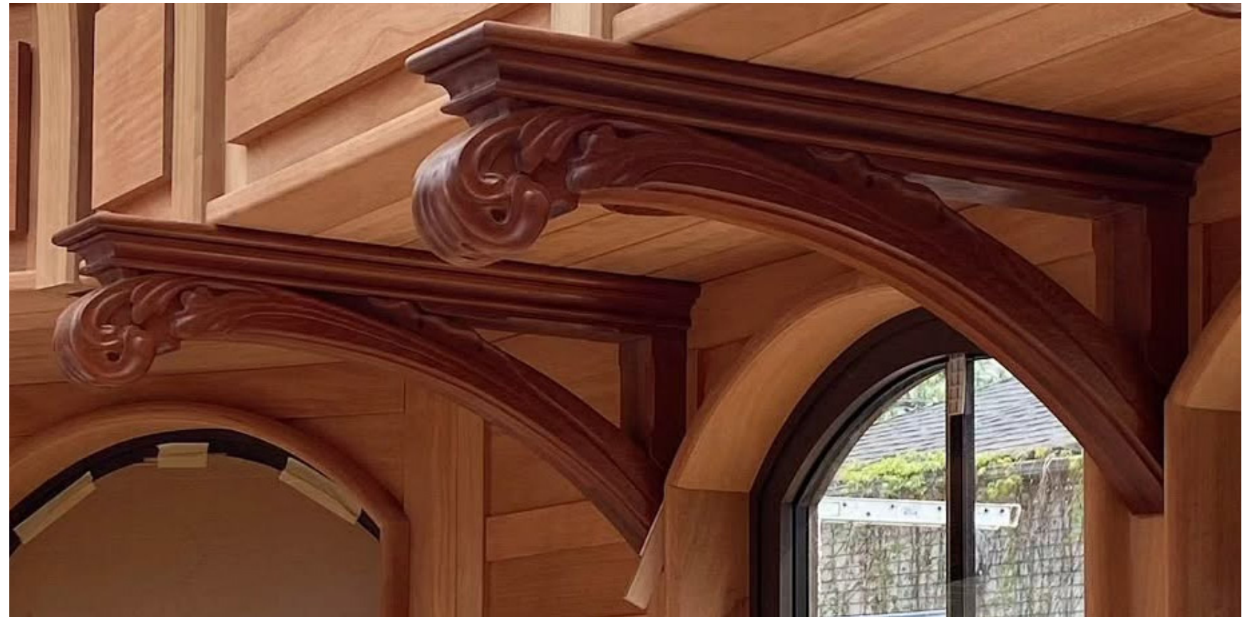
Mokeeta: Commission by Kevin Showell Featuring Photogrammetry with Reality Capture, Sculpting Touch-ups in ZBrush 3D Modeling/Compositing in Rhino and Toolpathing in RhinoCAM
